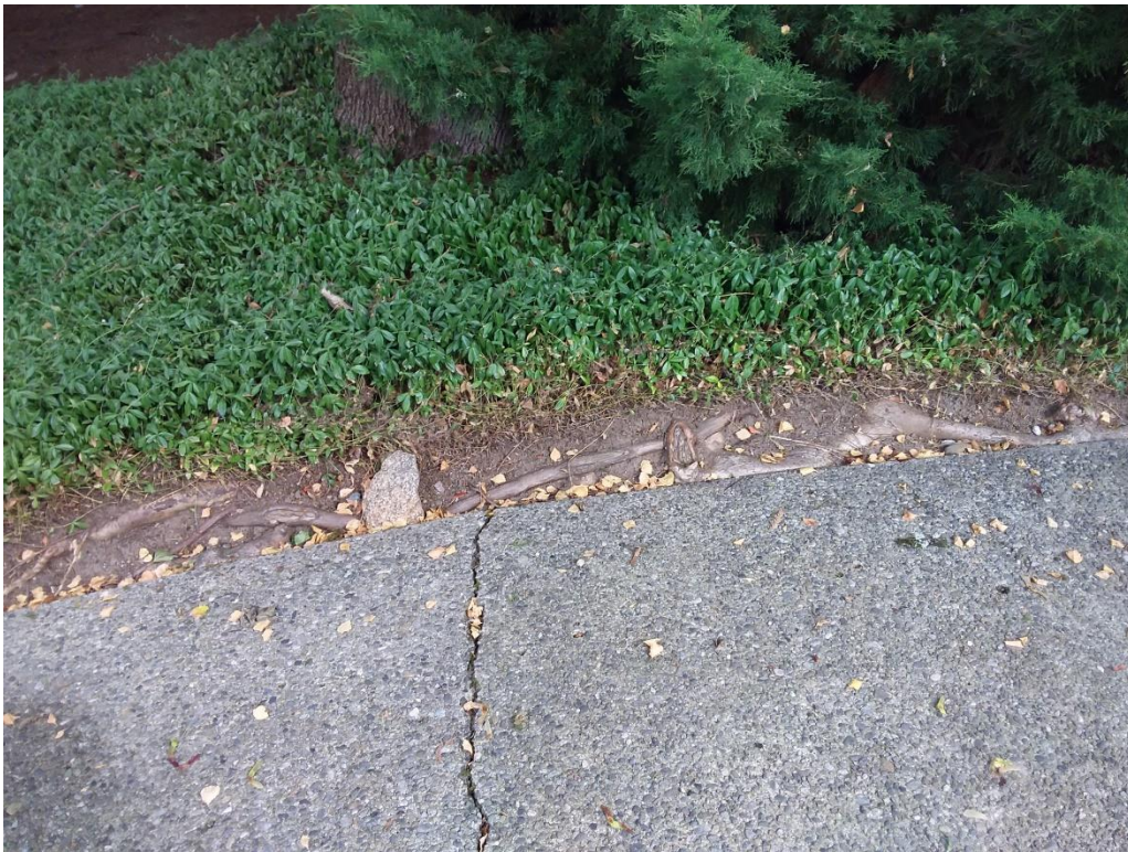
Figure 5. Looking down and north at the roots from the #581 maple growing along the north edge of the existing driveway.
